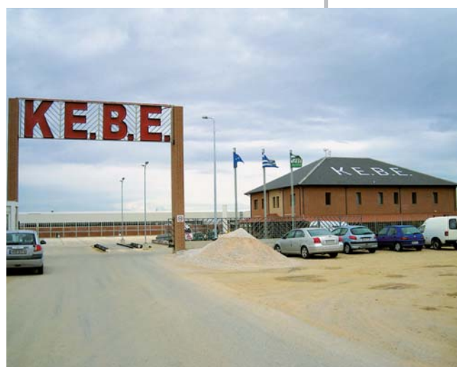
L'impianto KE.B.E. The KE.B.E. production plant
